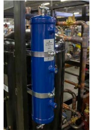
FIGURE 43: Oil Reservoir Check Valve (OCV)
