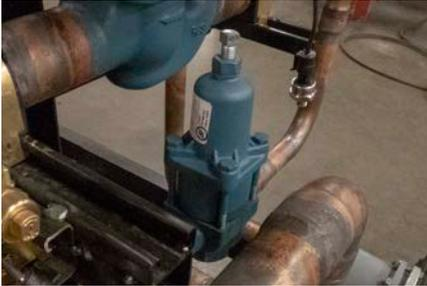
FIGURE 48: Electronic Pressure-Regulating Valve
