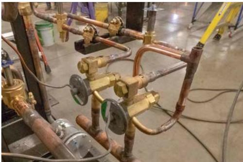
FIGURE 35: Electronic Expansion Valve (EEV)
