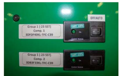
FIGURE 33: Defrost Control Module
