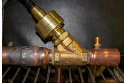
FIGURE 49: Pressure Transducer Valve
