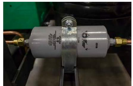
FIGURE 38: Replaceable Core Oil Filter
