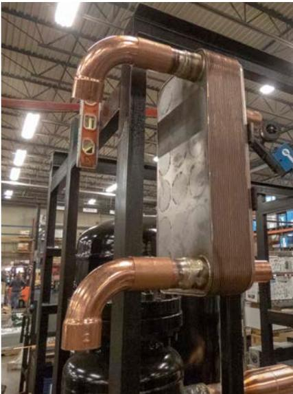
FIGURE 53: Subcooler/Heat Exchanger (Insulated)
