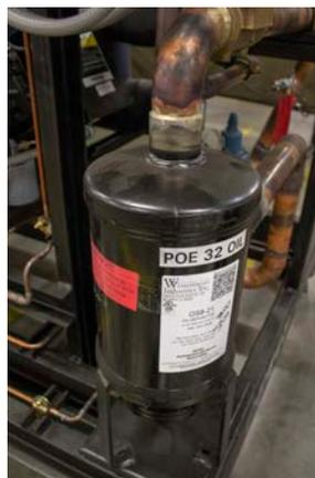
FIGURE 41: Impingement Oil Separator
