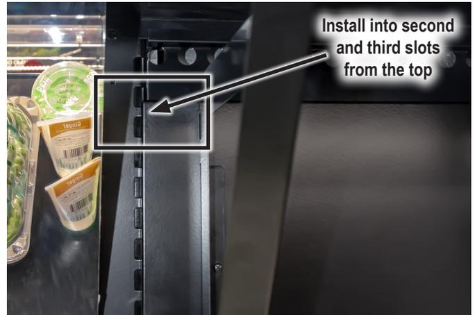
2. Install the mirror support into the shelf standards, using both the second and third slots from the top (See Figure 27 on page 15).
