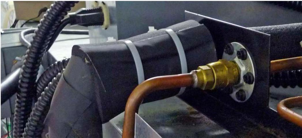
A pre-cut piece of split piping insulation (supplied) will be required on each freezer suction line quick-connect coupling. Cable ties will also be provided.
