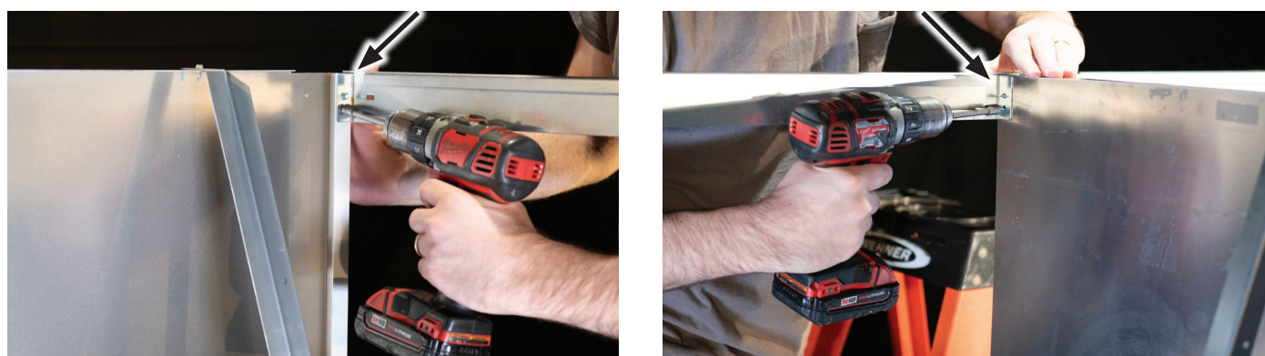
FIGURE 6: Mount the Signage Rail to the Side Shrouds
