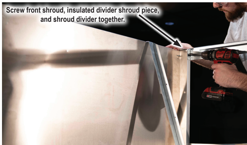
FIGURE 9: Install Insulated Divider Shroud Piece
