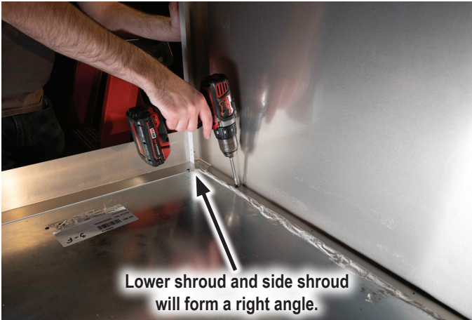
FIGURE 4: Screw Side Shrouds to the End Panel
