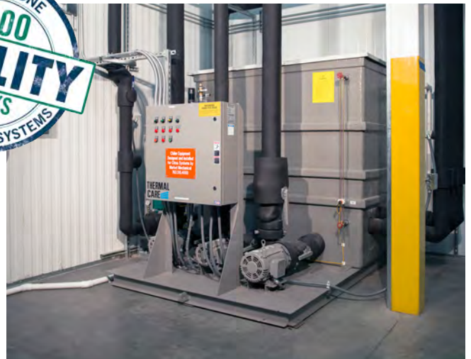
Chilled Glycol Pump Package
