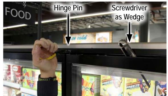
FIGURE 27: Push Door & Hinge Pin into Place
