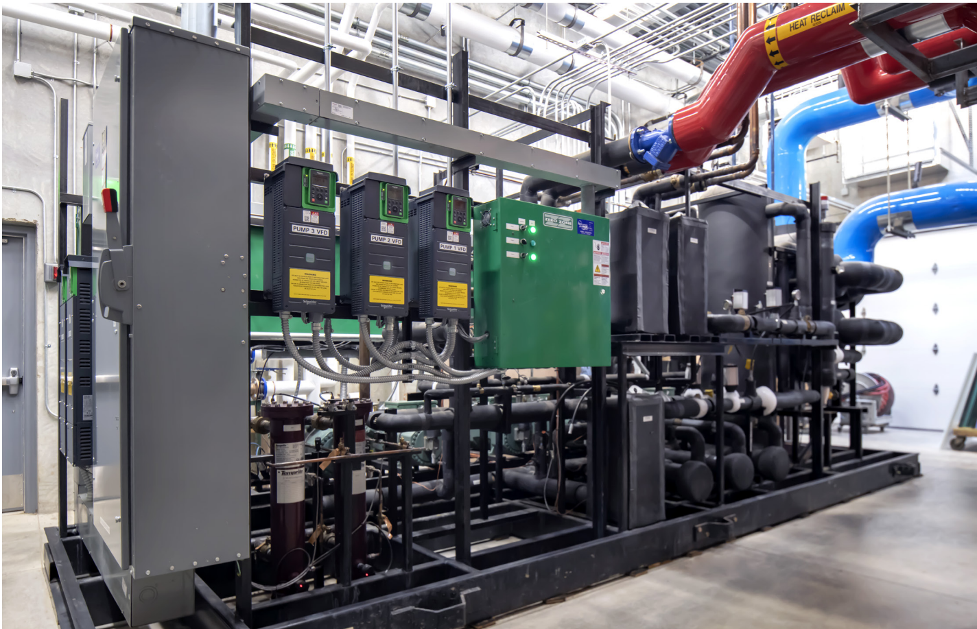
FIGURE 3: System 3 - CO 2 Packaged Chiller System
