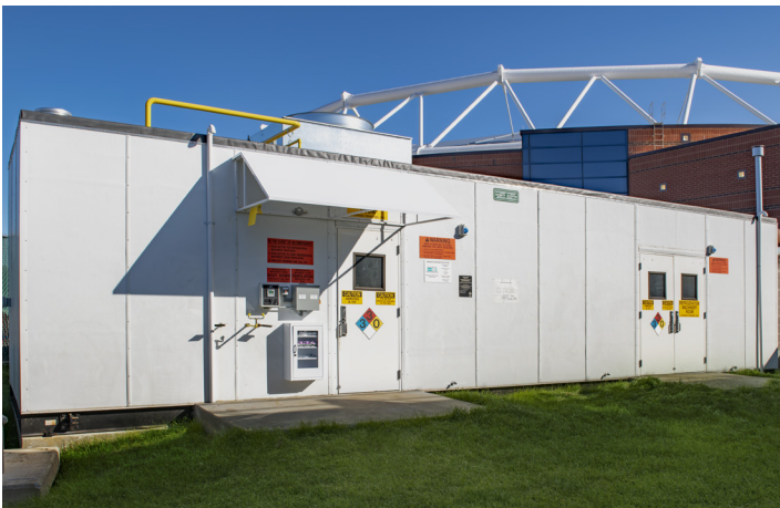
FIGURE 1A: System 1 - Ammonia Packaged Chiller Machinery Room, Exterior
