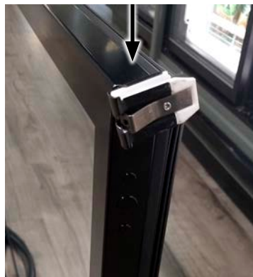
FIGURE 28: Remove Hinge Pin
