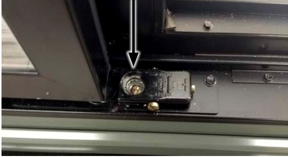
FIGURE 32: Torque Adjuster Locking Screw
