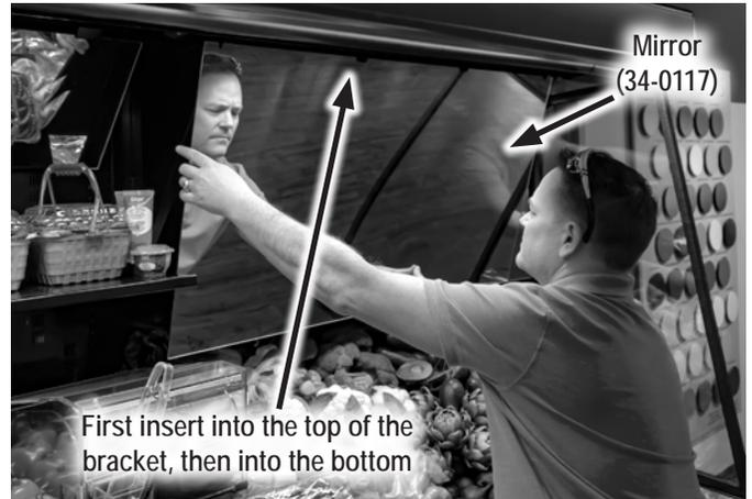
FIGURE 6: Mirror Installed and Centered
