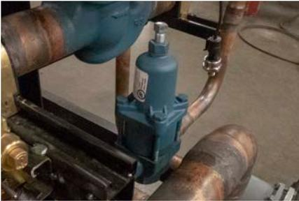
FIGURE 48: Electronic Pressure-Regulating Valve
