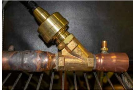
FIGURE 49: Pressure Transducer Valve
