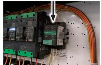
FIGURE 30: Control Relay
