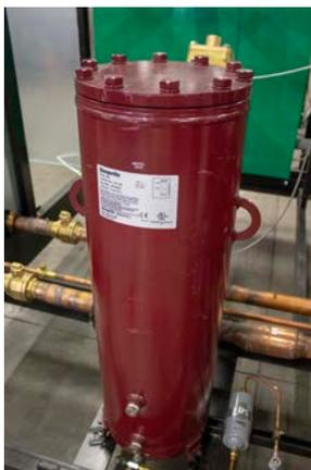
FIGURE 40: Helical Oil Separator
