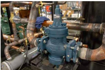
FIGURE 28: Liquid Differential Pressure Regulator (LDPR)
