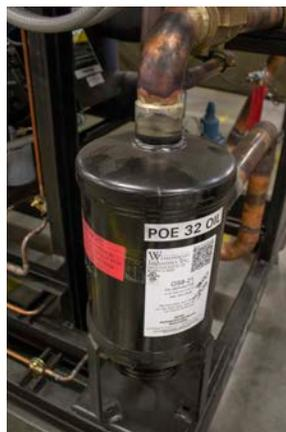
FIGURE 41: Impingement Oil Separator
