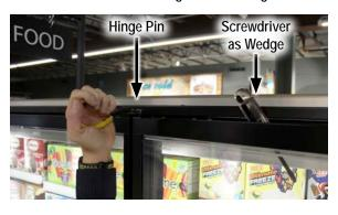
FIGURE 27: Push Door & Hinge Pin into Place
