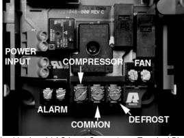
Fig. 11 - Load / AC Input Connectors- Terminal Blocks
