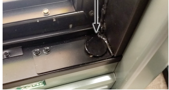
FIGURE 33: Torque Adjuster Plug
