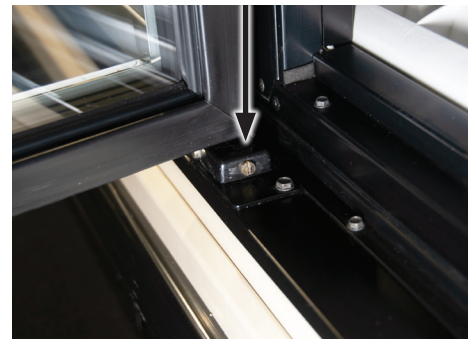
FIGURE 21: Sag Adjustment Screw
