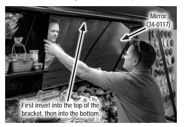
FIGURE 6: Mirror Installed and Centered
