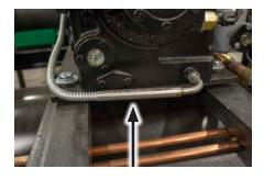
The **high-pressure control** shuts off a compressor when the discharge pressure of the compressor exceeds the set point. The **low-pressure control** ensures the compressor does not run in a vacuum. It can also be set to maintain a desired temperature in the refrigeration system.
