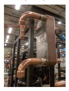
FIGURE 53: Subcooler/Heat Exchanger (Insulated)
