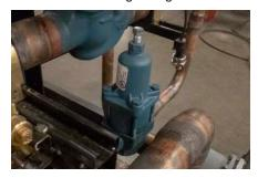
FIGURE 48: Electronic Pressure-Regulating Valve
