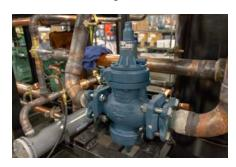
FIGURE 28: Liquid Differential Pressure Regulator (LDPR)
