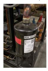
FIGURE 41: Impingement Oil Separator
