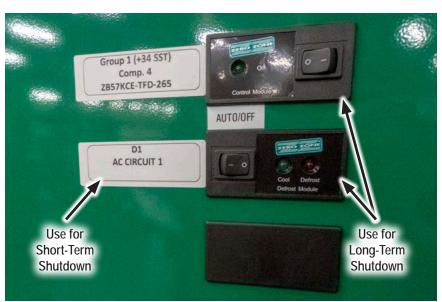
FIGURE 15: Control Switch and Circuit Switch
