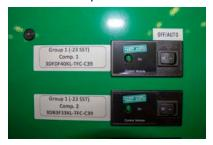
FIGURE 33: Defrost Control Module
