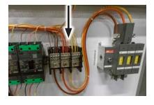
FIGURE 32: Compressor Control Module
