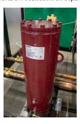
FIGURE 40: Helical Oil Separator
