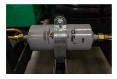
FIGURE 38: Replaceable Core Oil Filter
