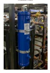
FIGURE 43: Oil Reservoir Check Valve (OCV)
