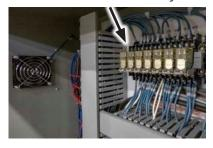
FIGURE 31: Power Distribution Block (PDB)
