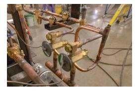
FIGURE 35: Electronic Expansion Valve (EEV)
