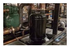
FIGURE 19: Horizontal Accumulator
