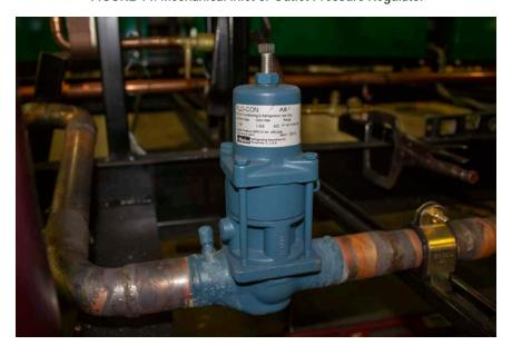
FIGURE 14: Mechanical Inlet or Outlet Pressure Regulator
