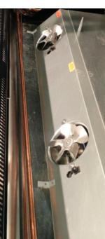
FIGURE 27: Fans and **Case-to-Case Piping**
