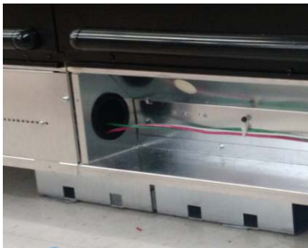
FIGURE 54: Case-to-Case Wiring
