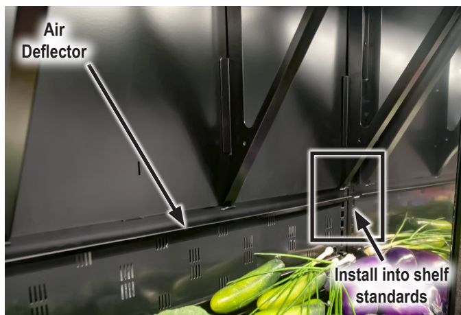
FIGURE 30: Install Air Deflector Under Mirror Support
