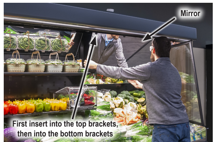
FIGURE 31: Hang the Mirror, Insert Top First
