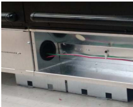
FIGURE 53: Case-to-Case Wiring
