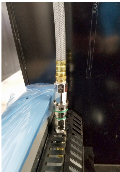
FIGURE 35: Spray Hose Connected
