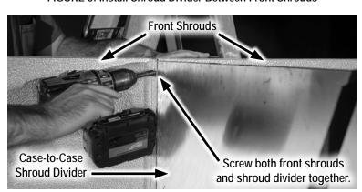
FIGURE 5: Install Shroud Divider Between Front Shrouds
