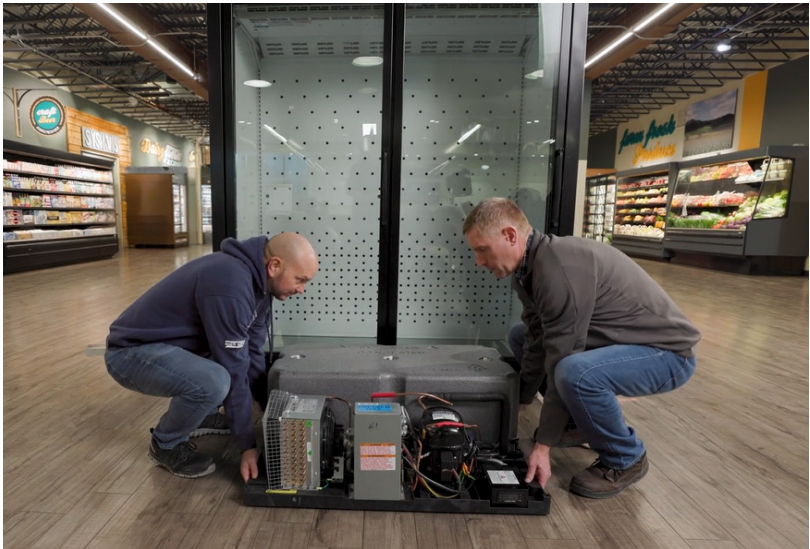
FIGURE 3: Lifting the PRU
