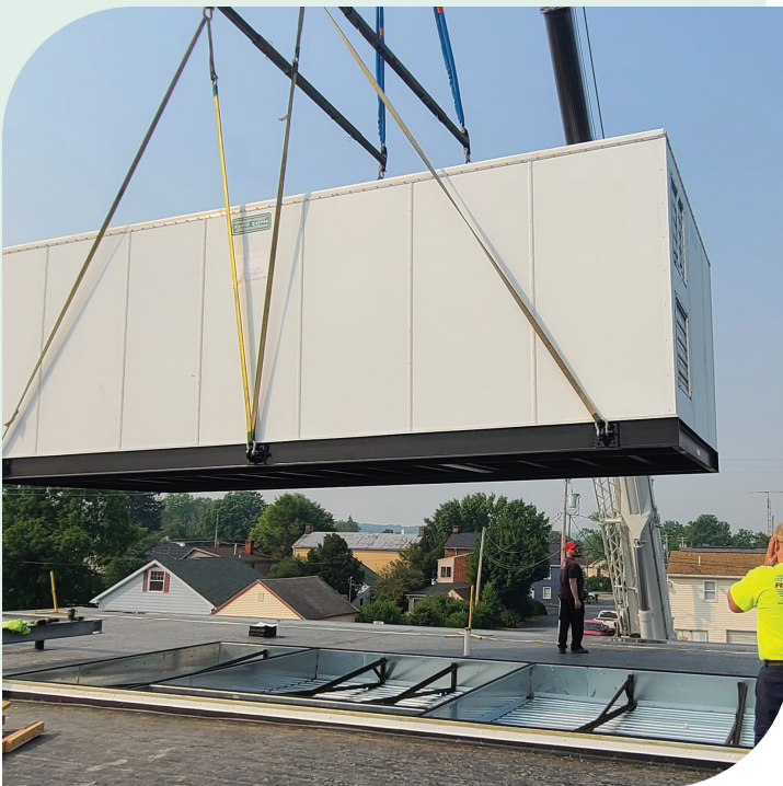
Installation of Custom Electrical Mechanical Center
