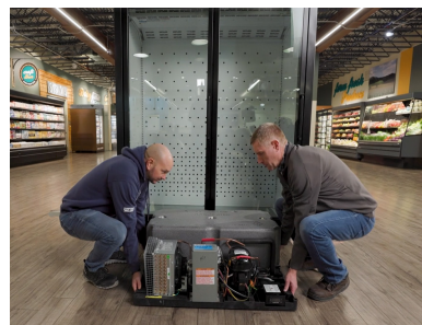
FIGURE 3: Lifting the PRU
