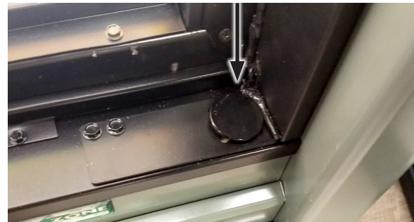
FIGURE 36: Torque Adjuster Plug
