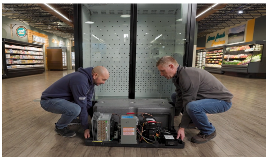
FIGURE 13: Lifting the PRU
