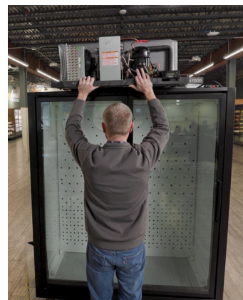
FIGURE 14: Aligning the PRU
